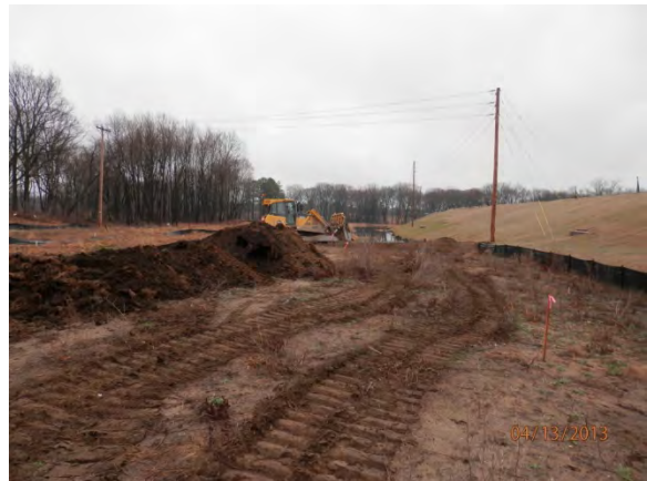
Photo 12. Stripping topsoil from area behind pump house.
