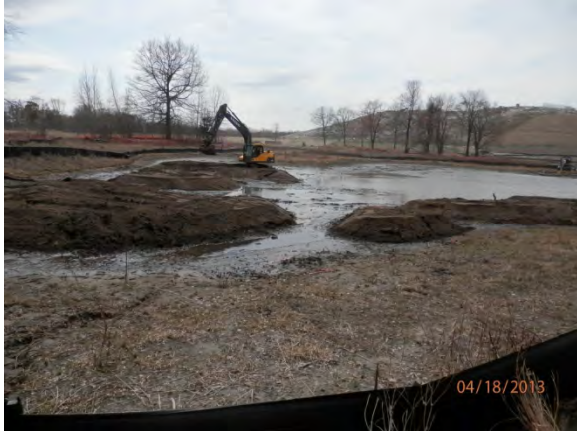
Photo 7. Construction of mounds in the north modified forested wetland area.
