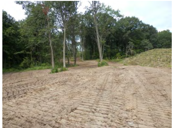
Photo 10. Areas U-5 in foreground and U-7 in background cleaned up, graded to previous contours and ready for seeding.
