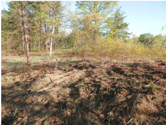
Photo 15. Area U-13 prior to grading to previous conditions.
