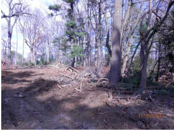
Photo 13. Area U-9 prior to tree thinning.
