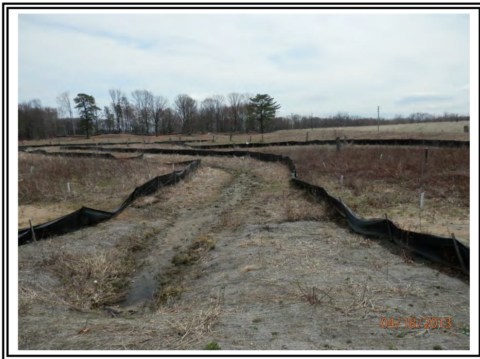
Photo 1- North Stream looking east from culvert in April.
