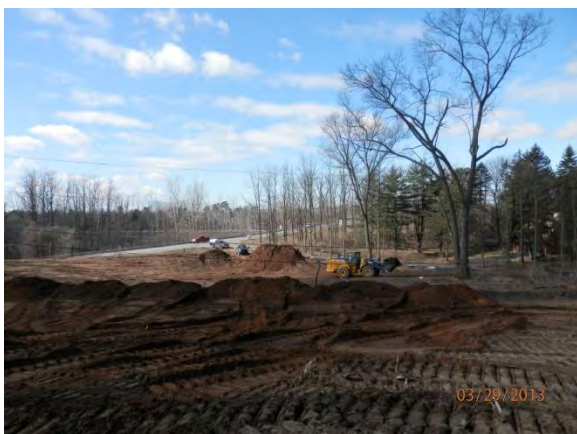
Photo 5. Stripping and stockpiling topsoil in area U-2.
