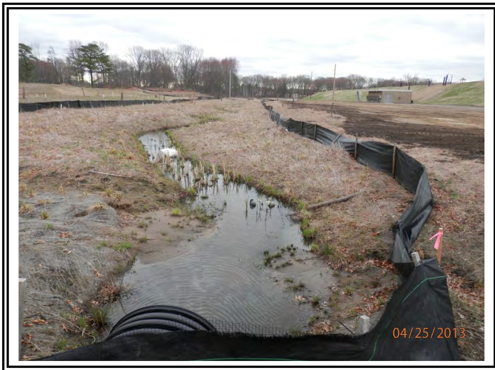
Photo 9- South stream looking east in April.
