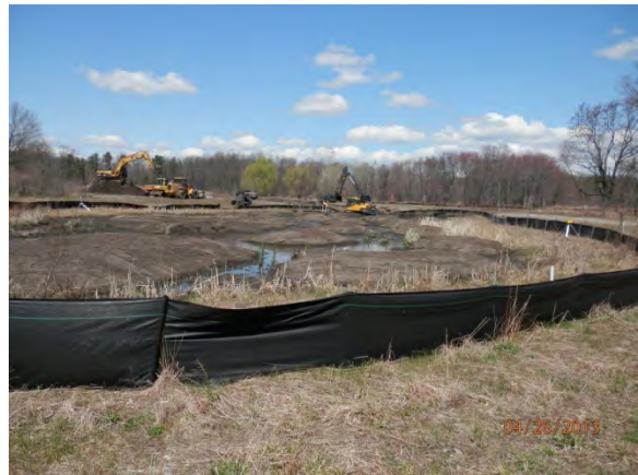
Photo 10. Construction of the mounds located in the south modified forested wetland area.
