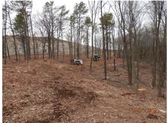
Photo 2. Clean-up activities in area U-1.
