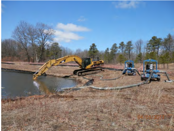
Photo 1. Pumping water from Vernal Pond.
