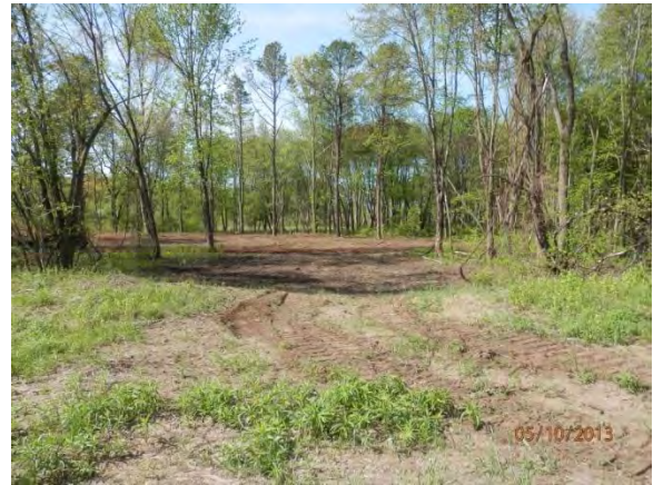
Photo 16. Area U-13 after grading.
