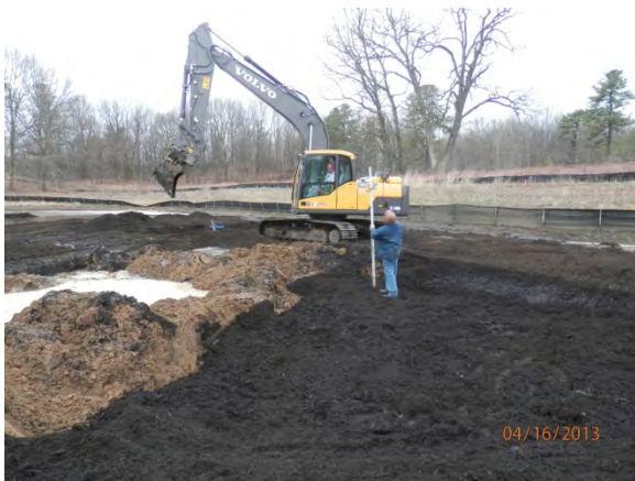
Photo 5. Checking grades of vernal pool.
