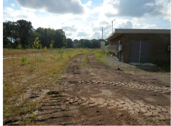
Photo 14. Conditions of area behind pump house on August 19, 2013.
