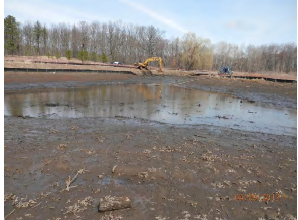
Photo 2. Final water drawdown for seining activities and to begin the placement of sand.
