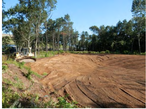
Photo 8. Softening of slope between U-1 and U-2.
