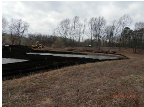
Photo 4. Placing compost and constructing pool areas.
